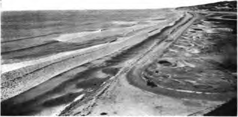
Before construction—a sandy, unkempt stretch of road.
